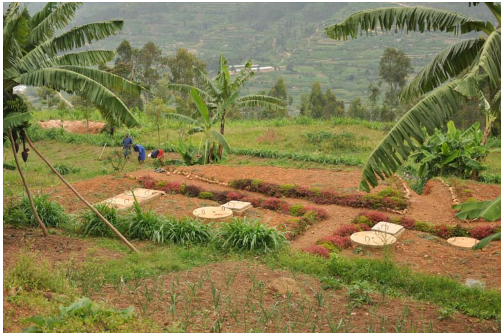
Figure 4.5: Biogas Digesters at Rulindo High School
